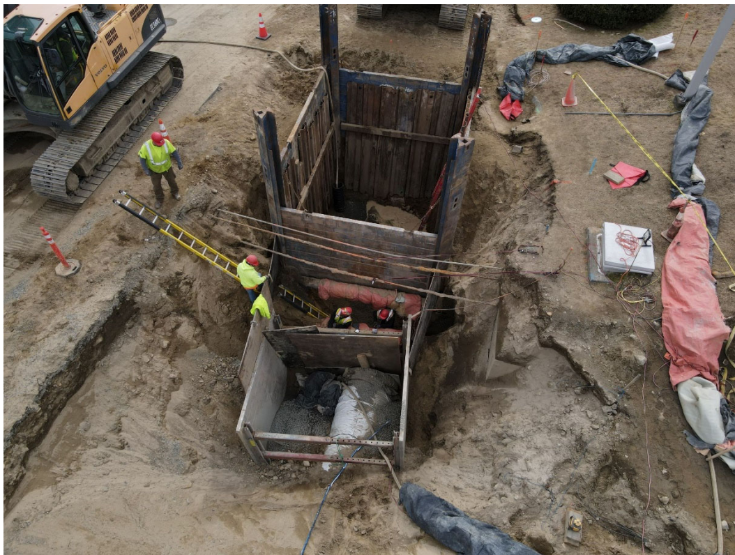
Installing 48-inch ductile iron backwash fill piping crossing existing piping conflicts
