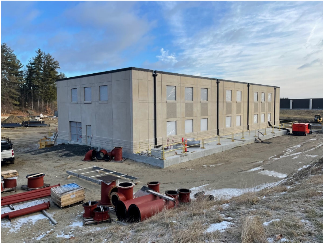
Backwash Pump Station Structure (over Clearwell)
