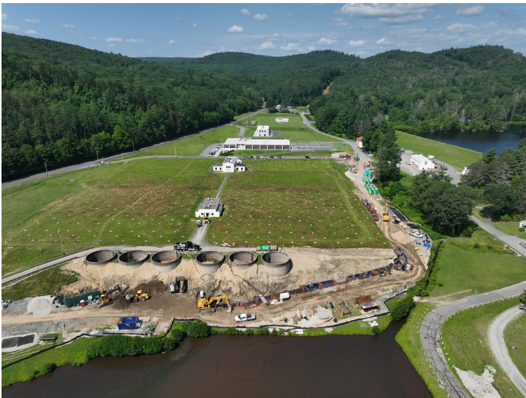
Construction of 36-inch HDPE bypass around the SSFs (SWSC drone photo 07/03/2025)
