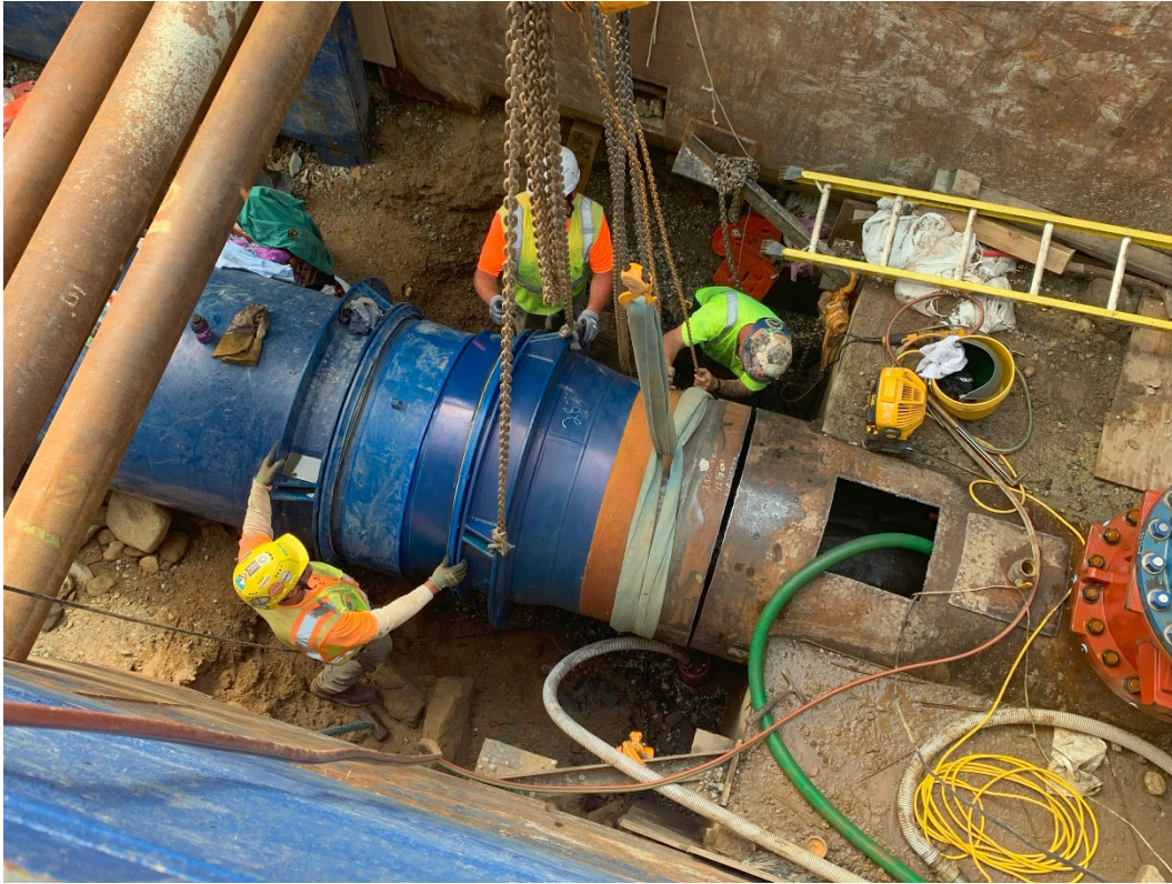
Installing final connections to new HDPE bypass (SWSC photo 08/15/2025)
