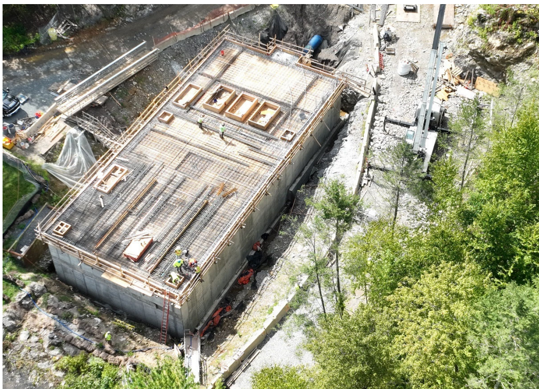
Roof slab reinforcement installation (SWSC drone photo, 09/08/2025)
