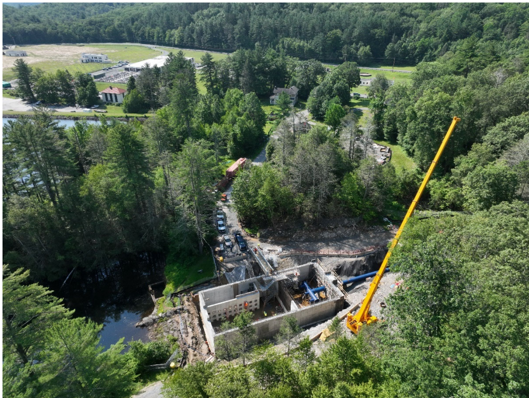
Construction of the EDV facility (SWSC drone photo, 07/03/2025)
