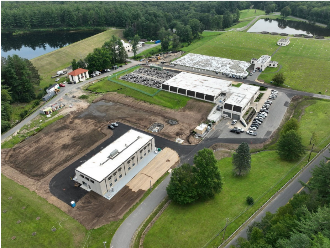
Backwash Pump Station & Clearwell Site, 08/10/23
