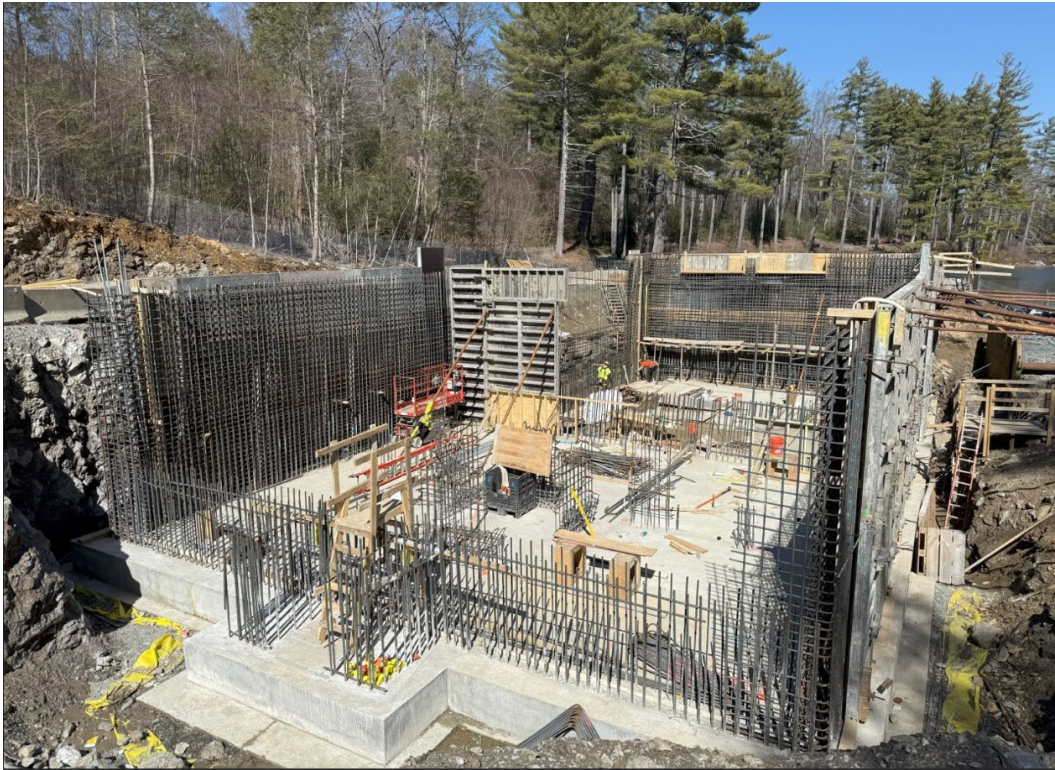
Installing rebar at EDV site (photo by AECOM, 03/19/2025)
