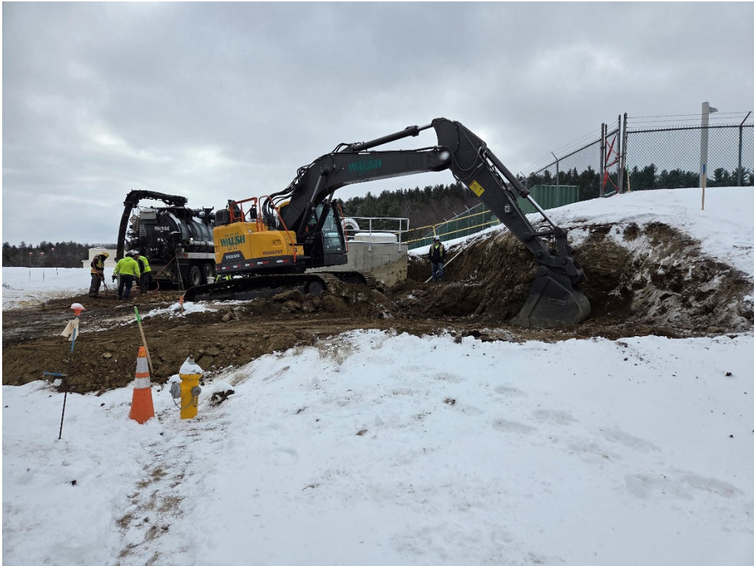
Breaking ground for transmission main relocations (photo by Hazen, 2/10/2025)
