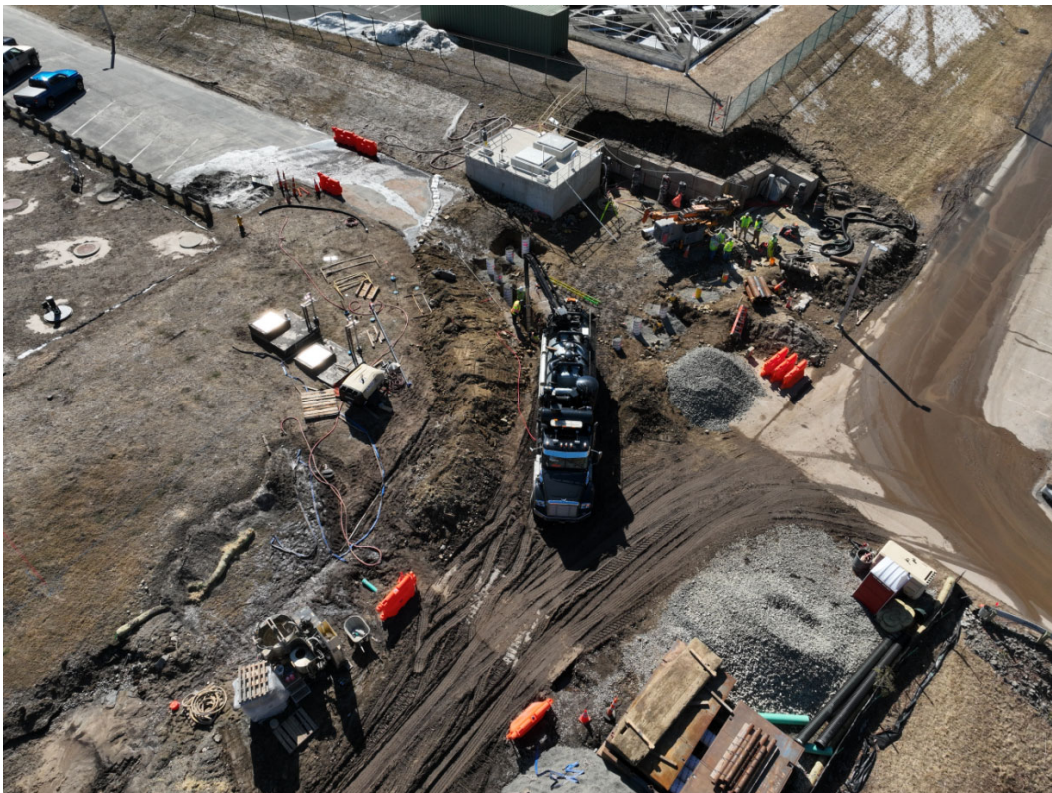
Excavating for transmission main relocations (SWSC drone photo 03/10/2025)
