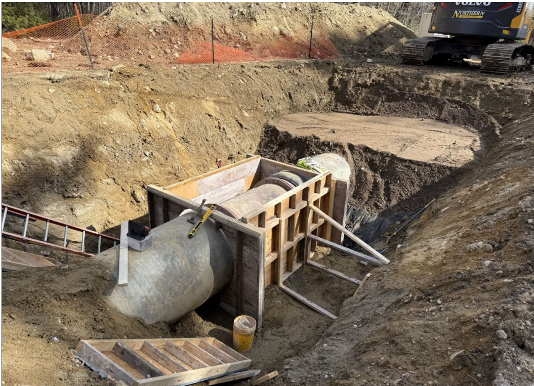
Replacing sections of PCCP pipe (photo by AECOM, 03/12/2025)
