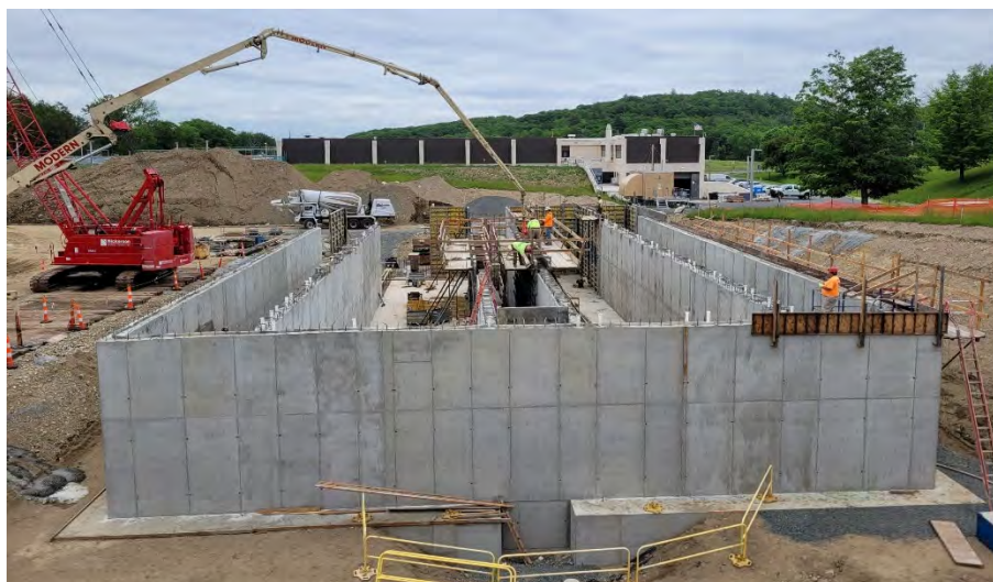
Construction of the new Clearwell structure
