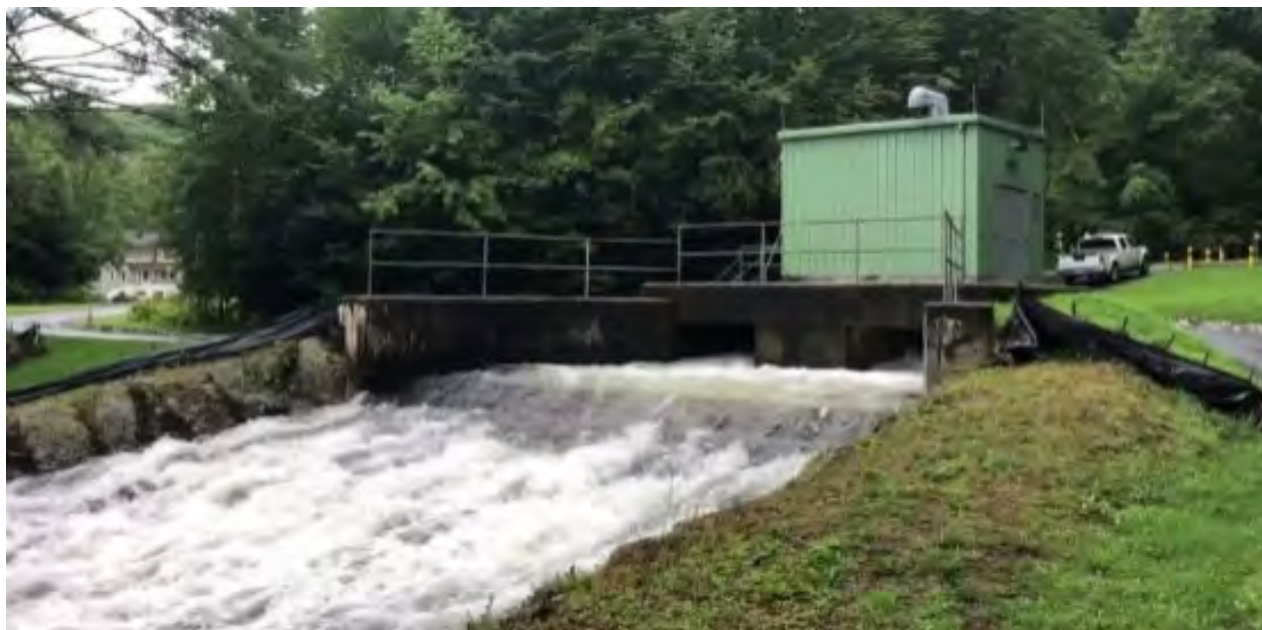
Outlet of the 42-inch bypass water supply main at the Sedimentation Basin
