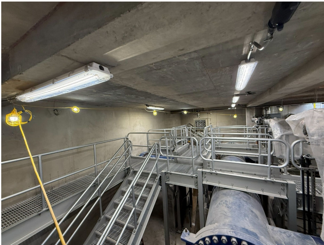
EDV Chamber interior (Engineer photo, 03/20/2026)
