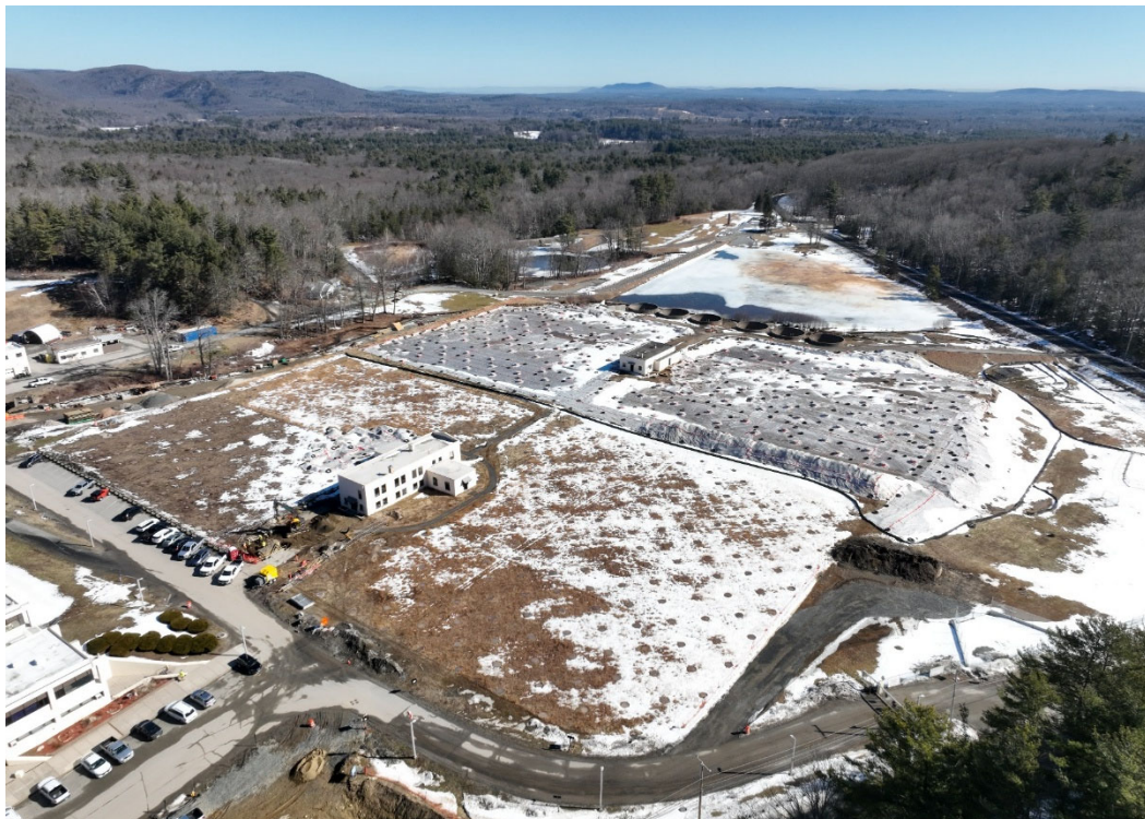
New WTP footprint and location of SSFs 7-10 and 15-18 (SWSC drone photo 03/10/2026)
