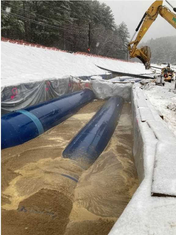
Backfilling 60-inch and 72-inch raw water pipes with flowable fill (L) and final backfill (R) (Engineer photo January 2026)
