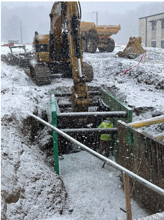
Installation of new drain (Engineer photo February 2026)
