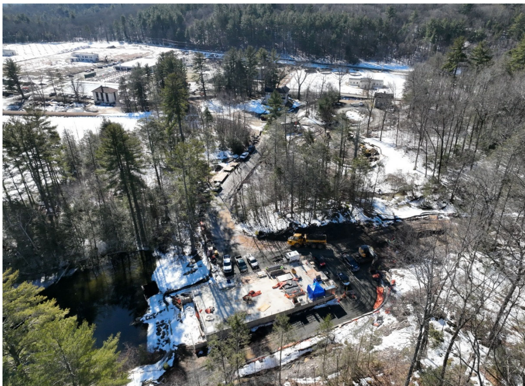
EDV facility site (SWSC drone photo, 03/10/2026)
