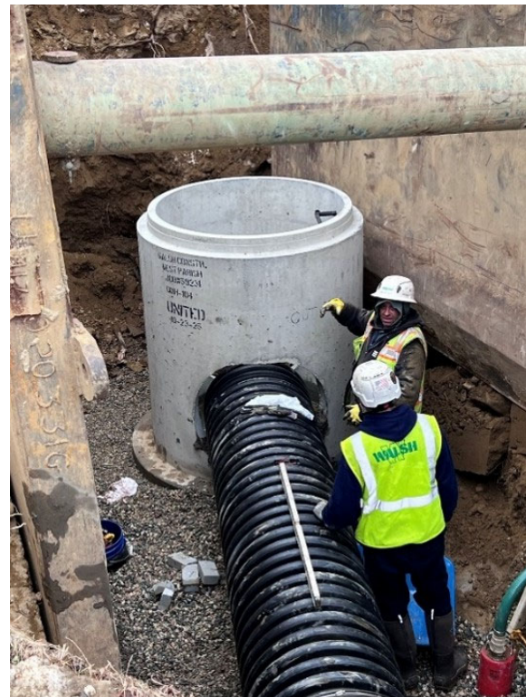
Installation of new drain (Engineer photo February 2026)
