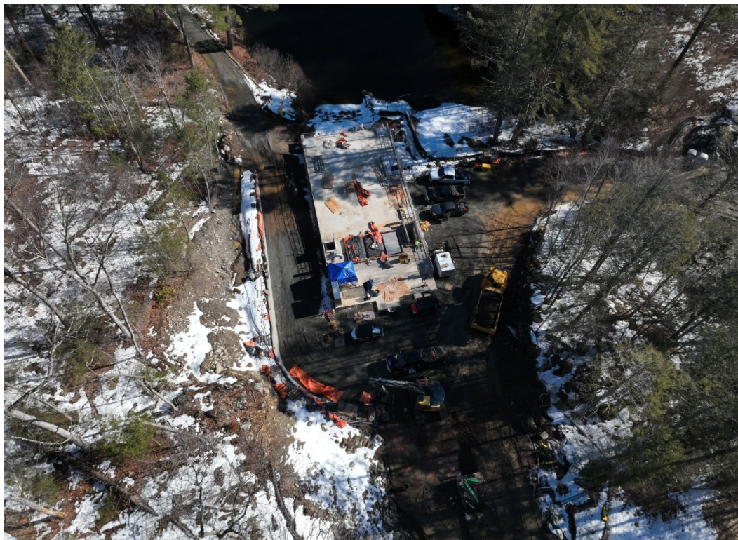
EDV facility site (SWSC drone photo, 03/10/2026)
