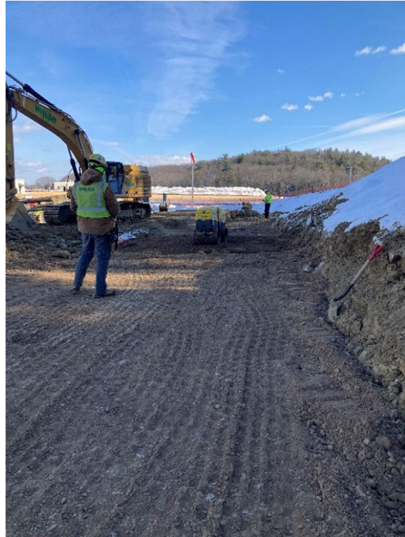
Backfilling 60-inch and 72-inch raw water pipes with flowable fill (L) and final backfill (R) (Engineer photo January 2026)
