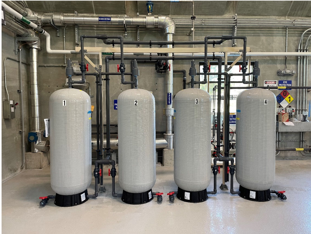
New mixing tanks installed on domestic water system, 05/07/2024
