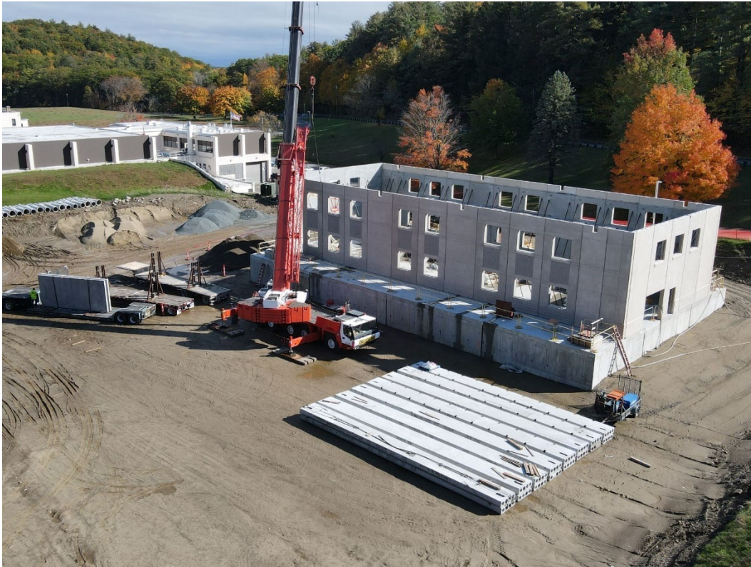
Erecting pump station precast concrete panels
