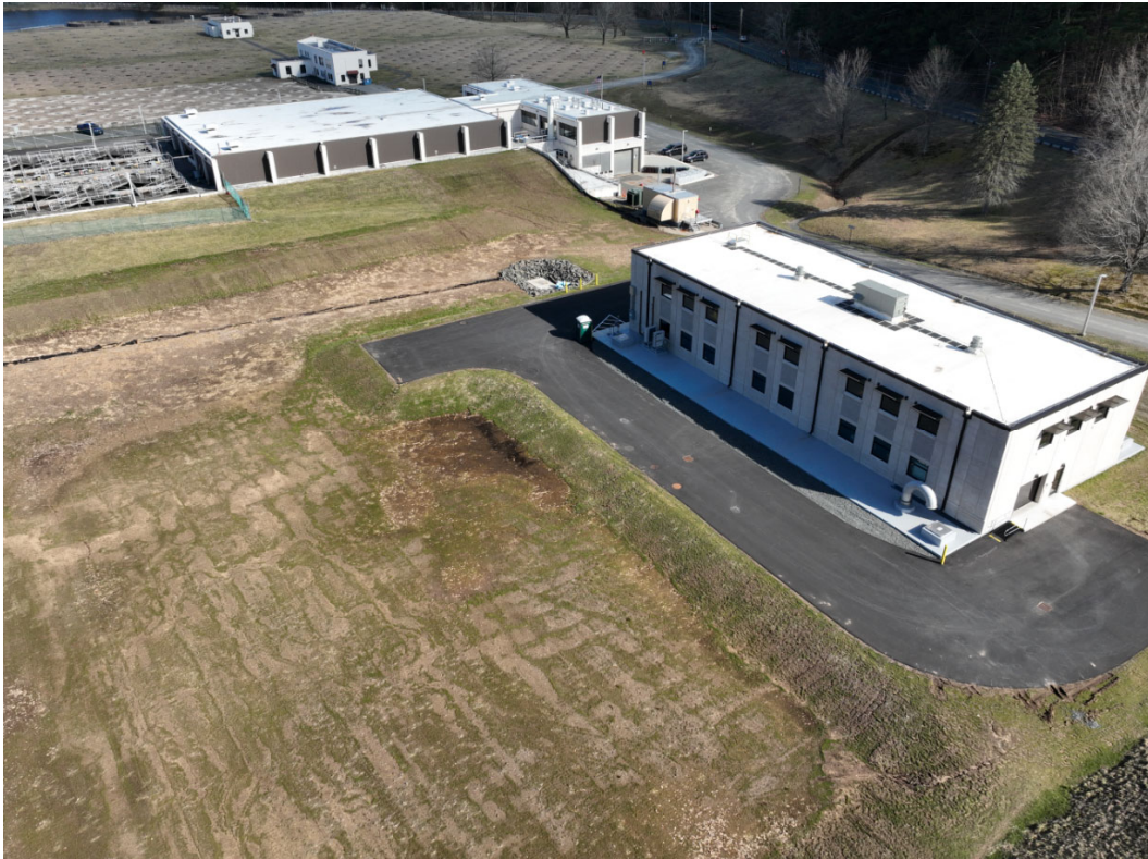
Backwash Pump Station & Clearwell Facility, 03/18/2024
