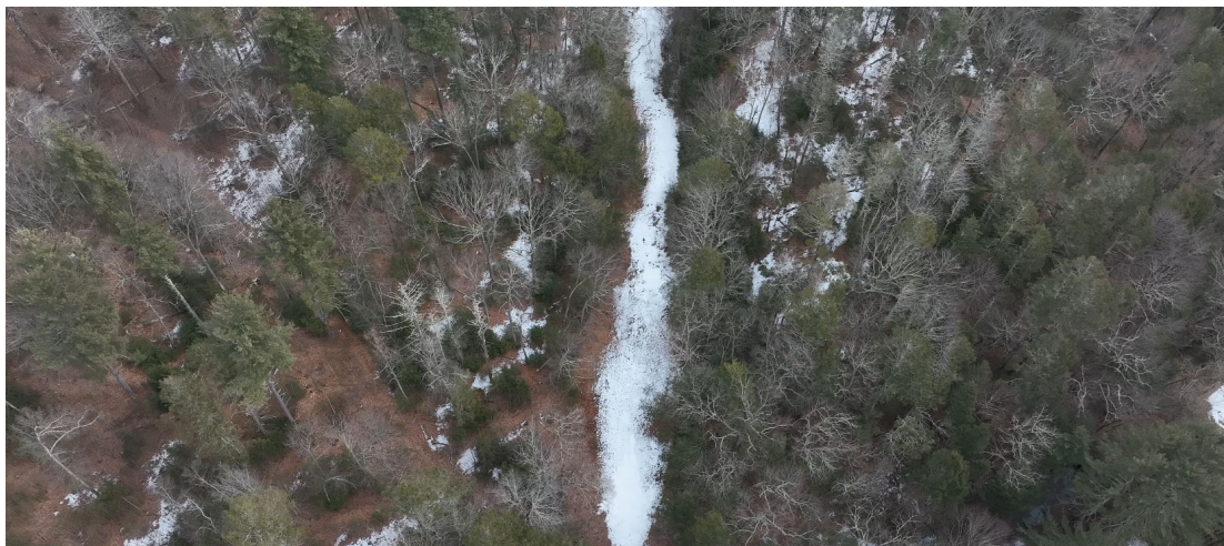
Drone footage of a section of the cross-country buried 42-inch pipeline, 02/22/2024
